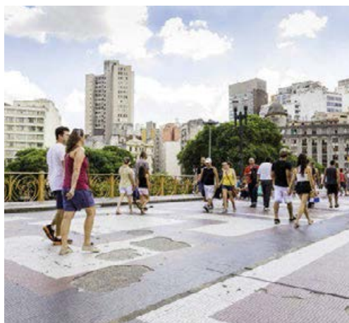
Santa Ifigenia viaduct, Sao Paulo, Brazil is marred by lack of maintenance © Frazao Production/Shutterstock.com
